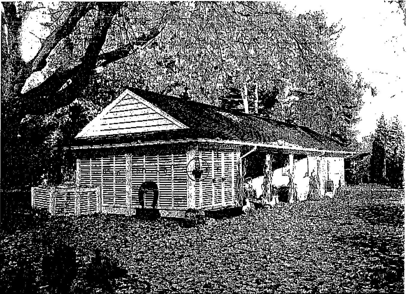
75. Toolhouse, southeast view
