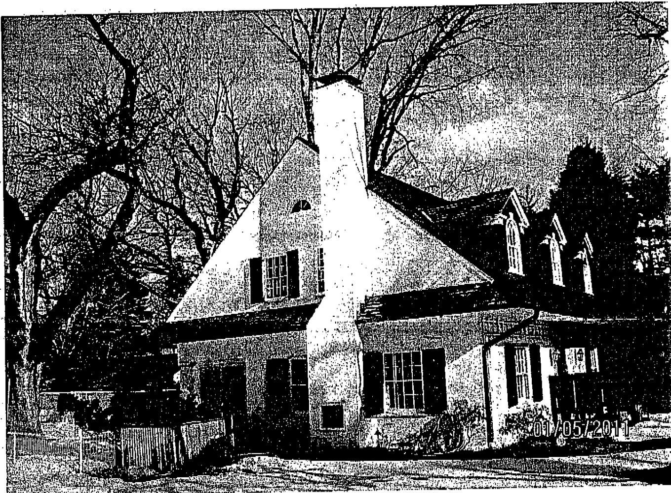
19. Cottage, southwest view
